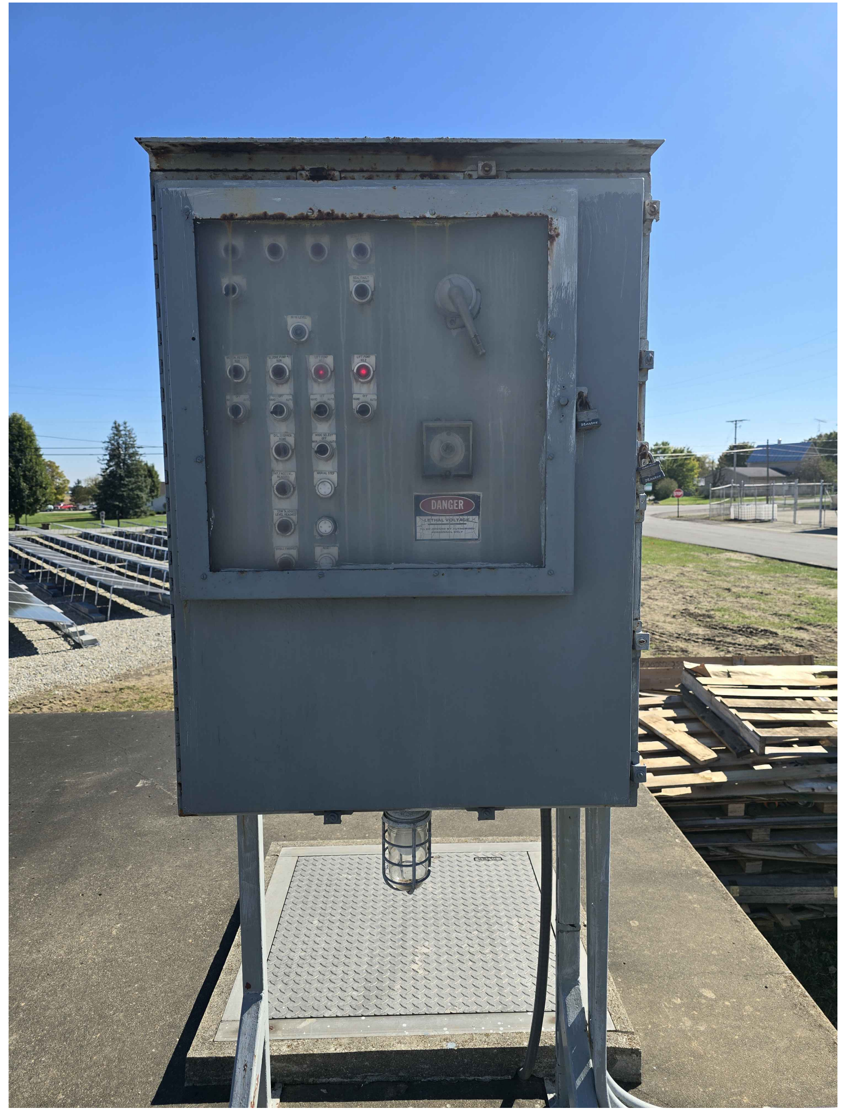
PHOTO OF EXISTING LIFT PUMP CONTROL PANEL
